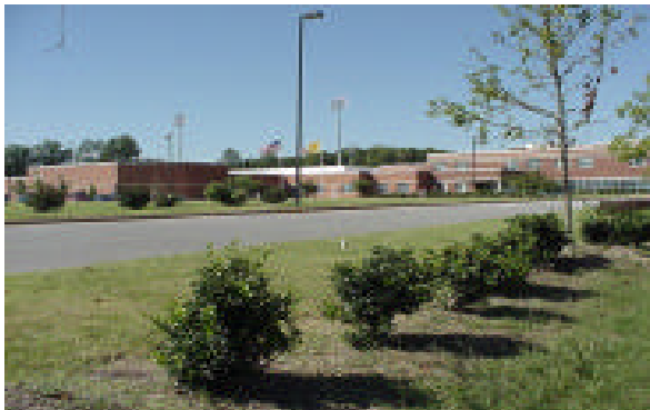
Main Campus on Edwards Mill Road
